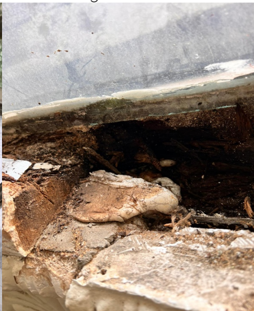
Photo 2 rotting out and silicone "blob"
